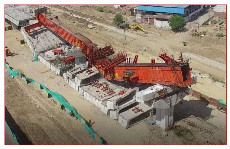
Cause of Failure – Poor Quality of Concrete & Segment Gluing operation
