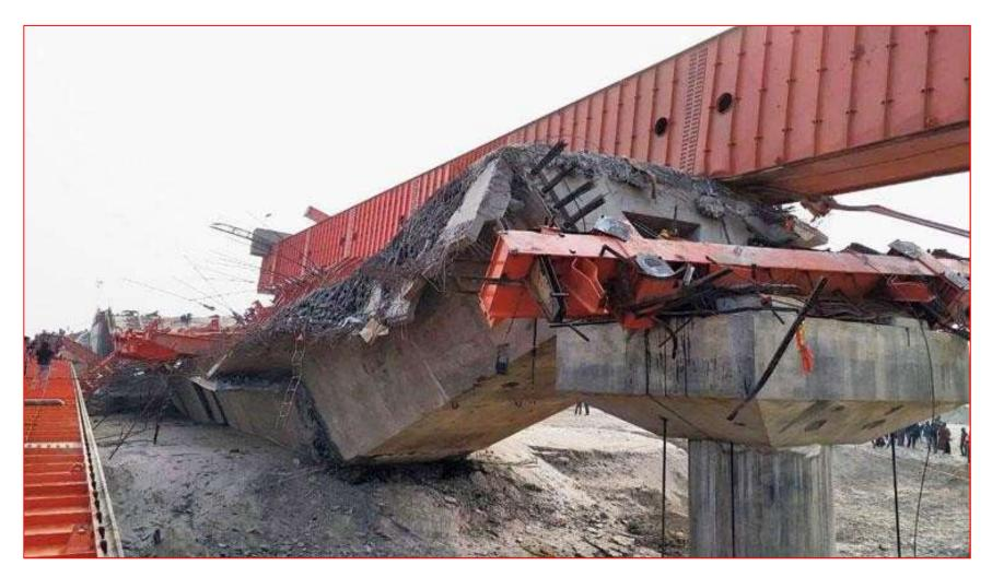
Cause of Failure – Launching girder failure
