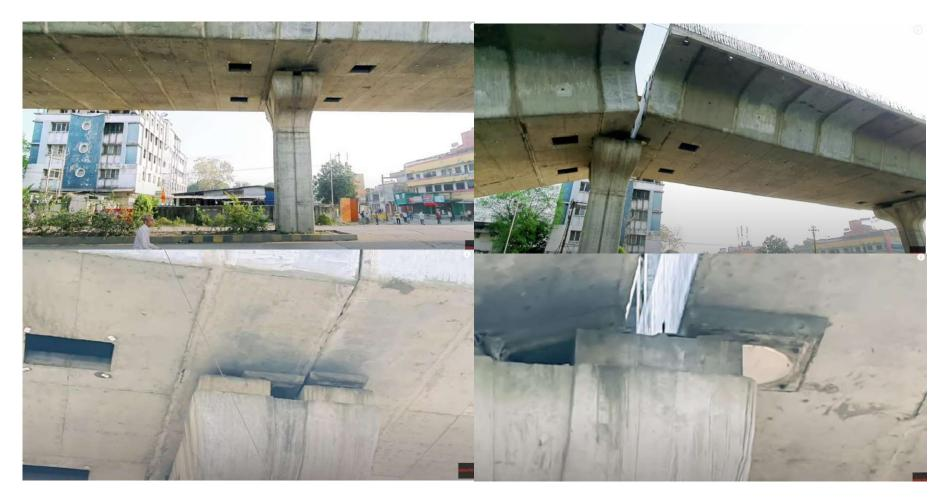
Cause of Failure – Incomplete Deck Continuity over a long time interval
