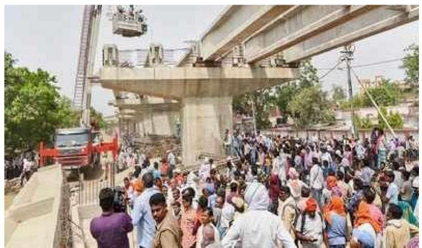
Cause of Failure – Inadequate Bracings in temporary condition & poor temporary supports
