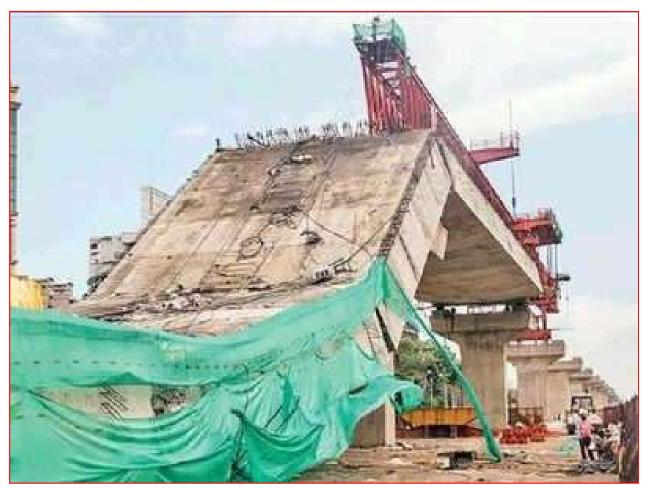
Cause of Failure – Poor Quality of Concrete & Segment Gluing operation
