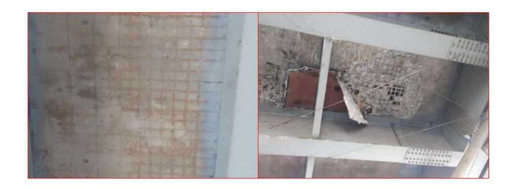
**Cause of Failure – Poor Quality of Concrete**
