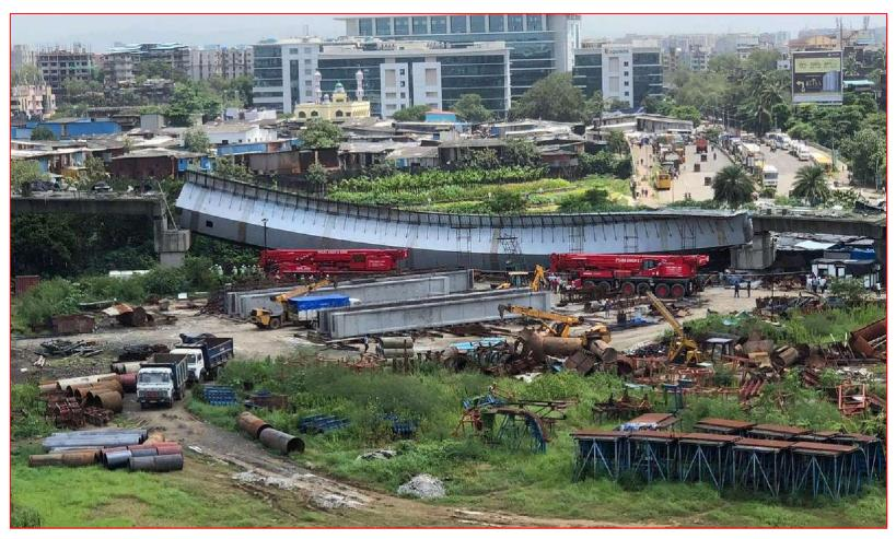
Cause of Failure – Inadequate temporary Support & poor temporary Bracings
