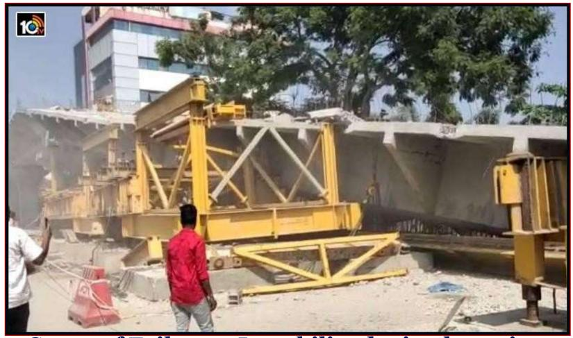
Cause of Failure – Instability during lowering operation
