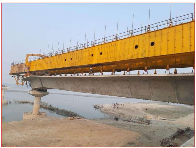
Cause of Failure – Poor Quality Segment Gluing operation/ Cable profiling
