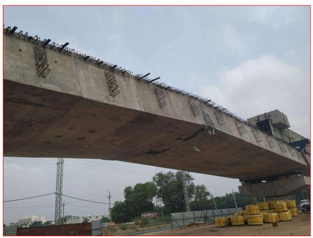
Cause of Failure – Poor Quality of Concrete & Segment Gluing operation
