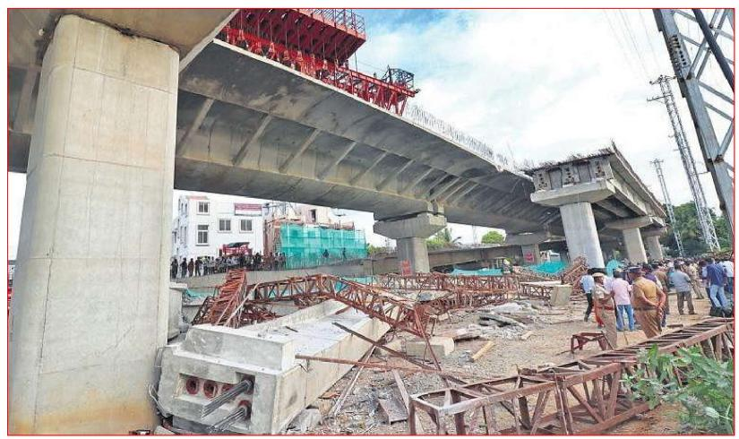
Cause of Failure – Inadequate Bracings in temporary condition & poor temporary supports
