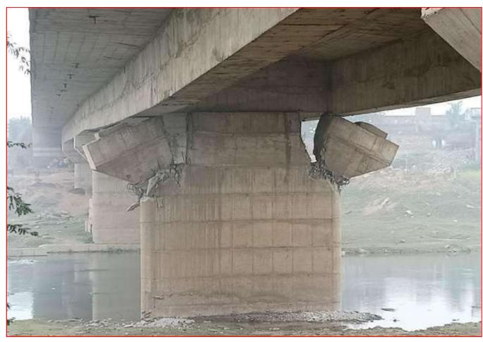
Cause of Failure – Improper Reinforcement Detailing and Incorrect Bearing Installation
