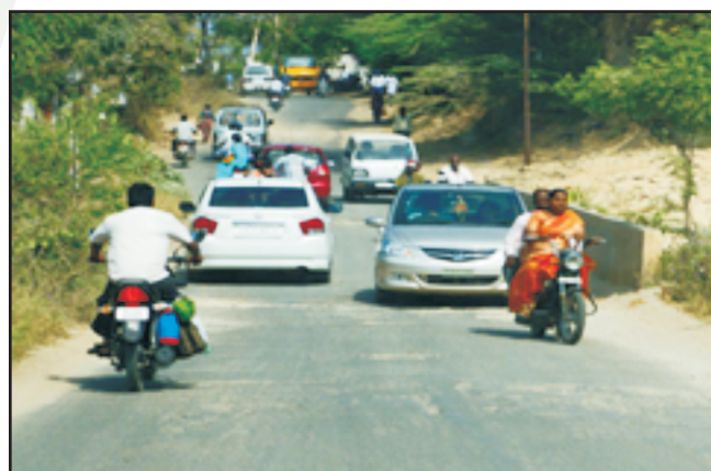
Photograph 3 – Narrow road width may provoke accidents during overtaking-A Safety Issue on PMGSY Roads
