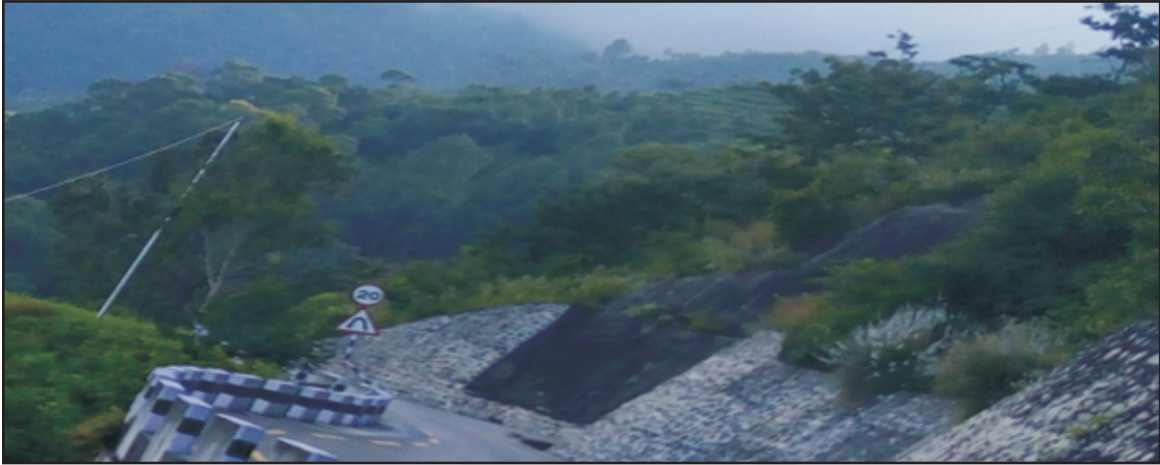
e) Rock bolting/Stabilization of slopes/fractured rocks by construction of RCC bands bolted with high tension steel cables
