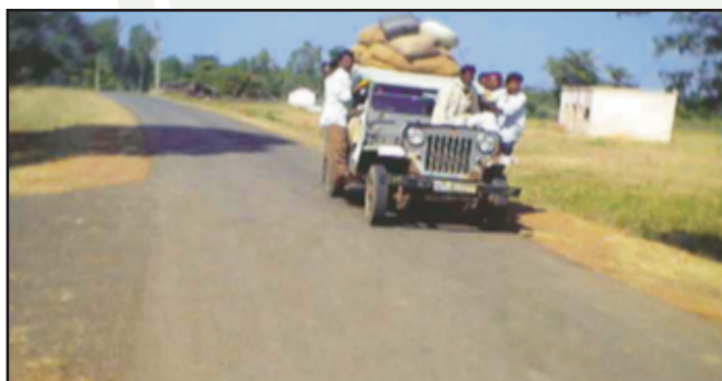
Photograph 2 - Overloading of Passenger Vehicles is another Safety Issue on PMGSY Roads
