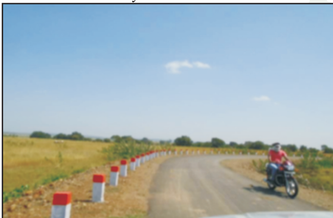
Photograph 6- Guard Stone provided at Sharp Curves enhances safety on PMGSY Roads
