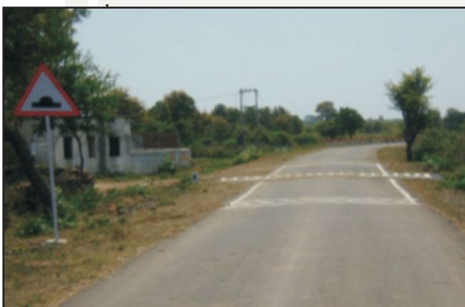
Photograph 7 –Provision of Road Humps near schools, Habitations etc. Enhances Safety
