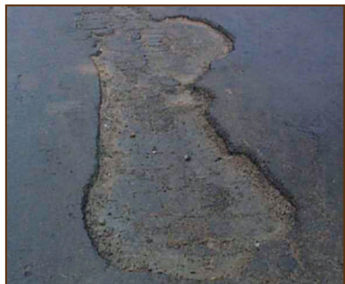
Figure 8: Delamination
