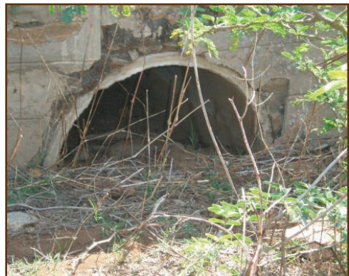
Figure 17: Blocked culvert
