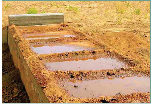
Figure 25: Creating a water pond for curing
