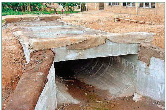
Figure 24: Curing of concrete with wet gunny sacking
