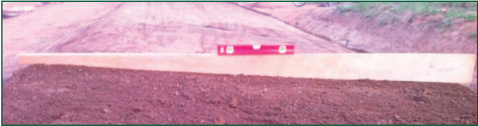
Figure 7: Checking camber with camber-board
